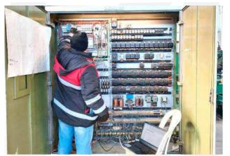
Our team fixed errors in the Gartemann & Hollmann control program based on the client's demands. Slave devices in the Profibus industrial network were deactivated during the work, along with the software functional block that debugged the automatic servo control and the block that calculated time intervals, the mark's speed of movement, the servo drive's current rotation speed, and the block that handled the human-machine interface.
